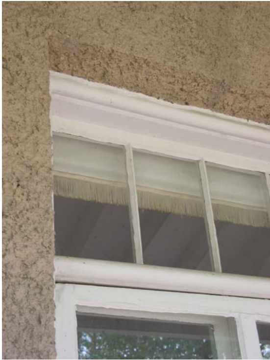
Figure 5: Rectangular windowpanes along the roughcast south façade of 19 Jason Road
