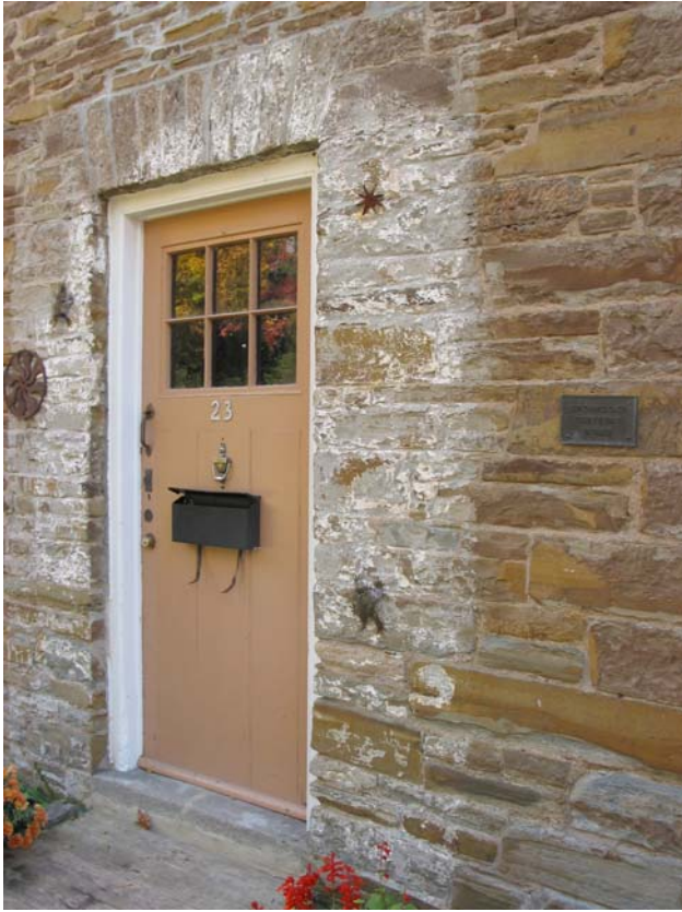
Figure 3: Main entrance of 23 Jason Road
